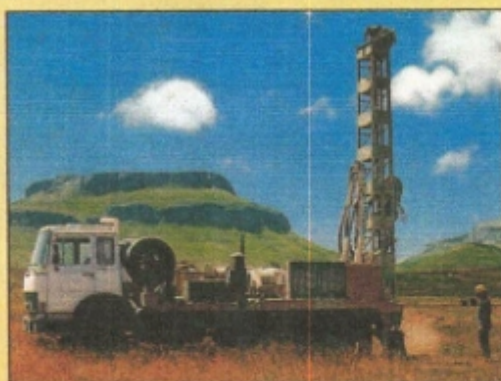
Heavy weight drilling rig, type P 5001
